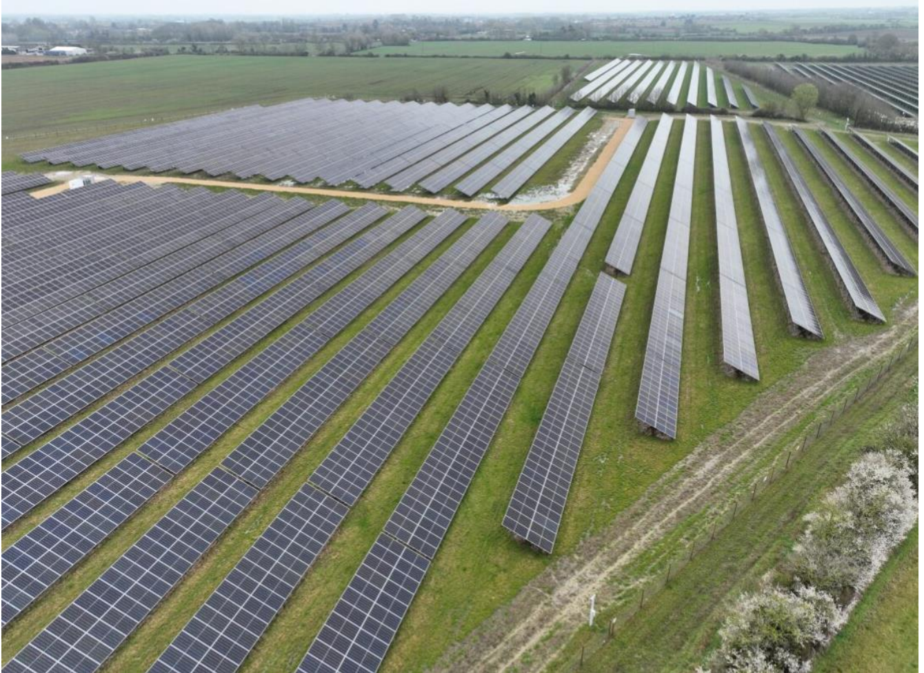
Plate 1: Typical Solar Panels
