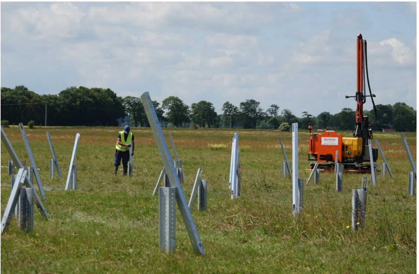
Plate 6: Example of a piling rig and piles
